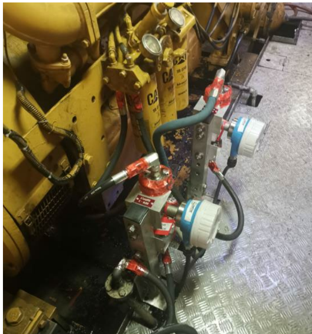
Figure 3.34 – Flowmeters connected to engine (Source: Bourbon Marine & Logistics)
