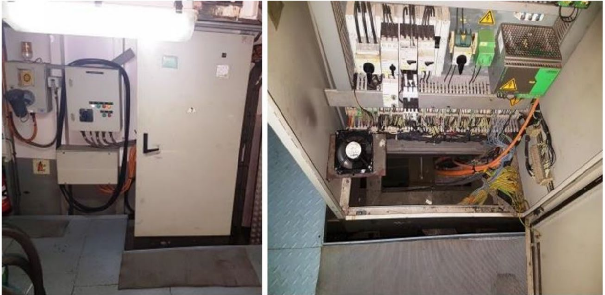
Figure 3.7 – Electrical Cabinets in Z-Drive compartment ( Bourbon Rhesos , 2019) (Source: Bourbon Marine & Logistics)
