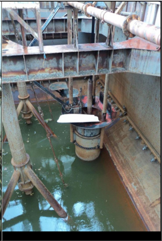
Figure 3.12 - Overturned boat on fore overflow (Source: Operator)
