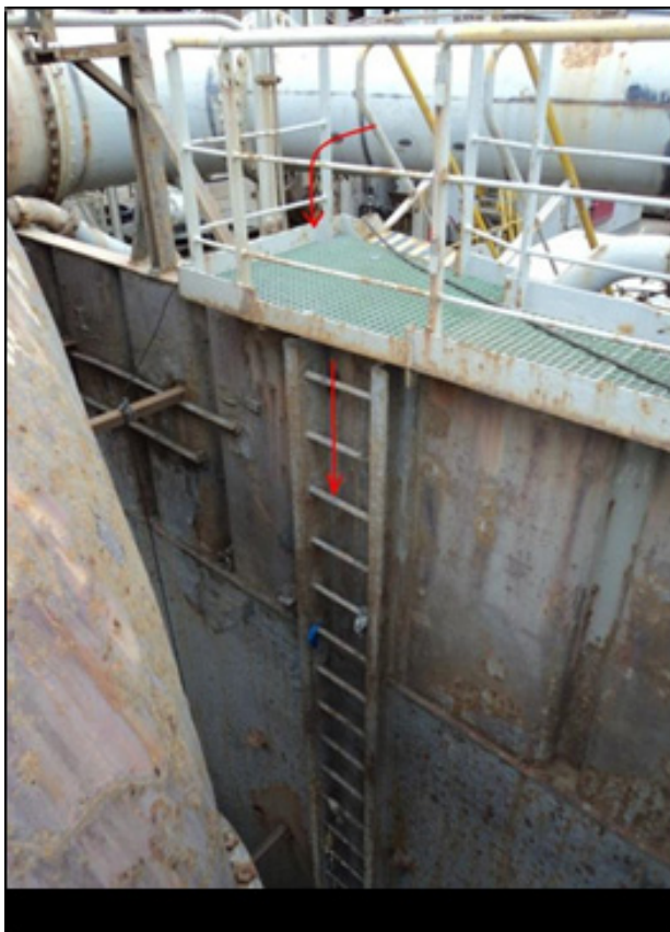
Figure 3.3 - Aft 'Out-of-use' Ladder into hopper (Source: Operator)
