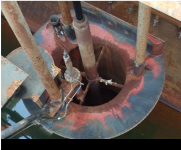
Figure 3.1 - Fore Overflow (Source: Operator)
