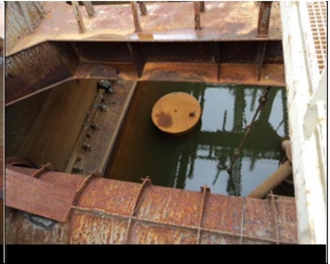
Figure 3.2 - Blinded Aft Overflow (Source: Operator)
